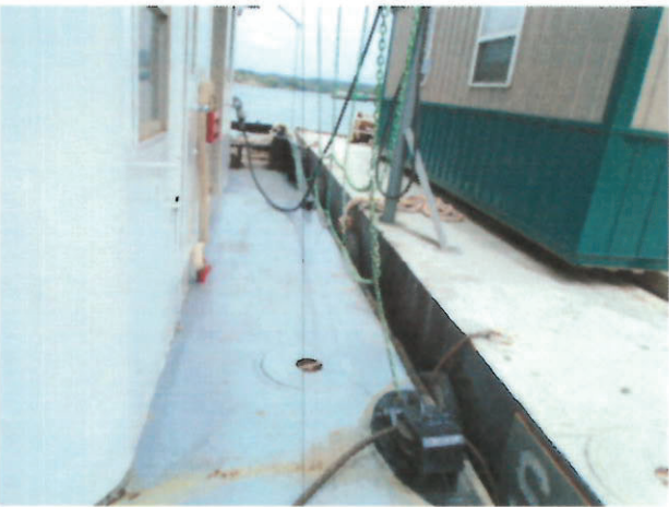
Port side deck looking aft
