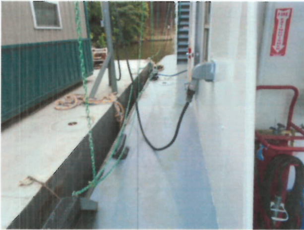
Starboard side deck looking forward
